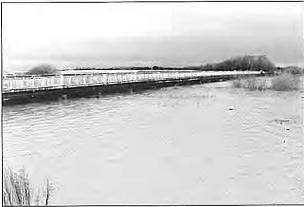
State Highway 2 Waitangi Bridge July 1992
