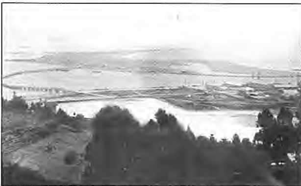
View over Napier in 1880 - Bridge at low tide. Much of Aburiri and Westshore is built on alluvial deposits. (Photo courtesy of Don Wilkie collection)
