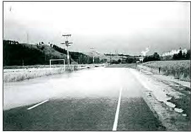
Flooding from Esk River on State Highway 2 March 1987.
