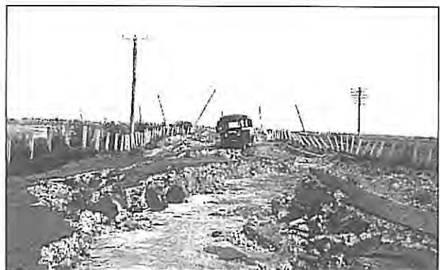
Bus stranded on crumbled road near Poukawa 1931. Fence line and power poles have buckled along the road due to intense shaking. (Photo Institute of Geological and Nuclear Sciences)
