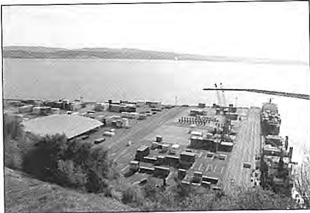
No 5 Kirkpatrick Wharf Port of Napier July 2001. (Photo courtesy HBRC)
