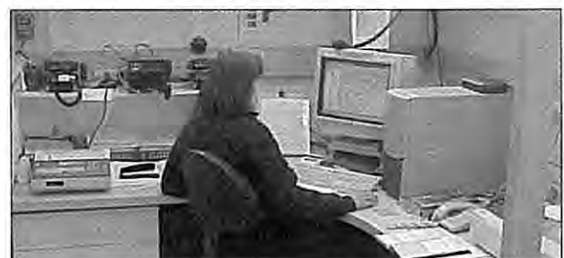
Telemetry room at the Hawke's Bay Regional Council October 2001.
