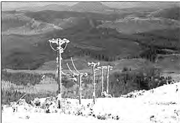
Power Lines feeding power to TeWaka have had their spans shortened by including extra poles. This was necessary to prevent the combination of ice and wind causing the spans to collapse under the strain. (Photo courtesy Ian Greaves Telecom)
