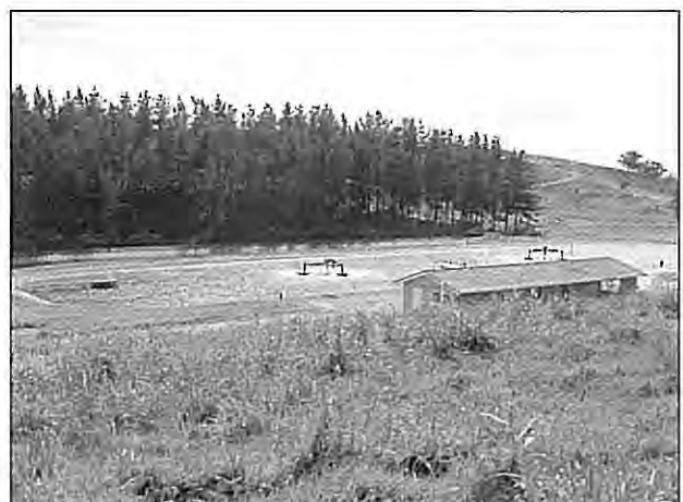
Wairoa wastewater plant aeration lagoon and control building. (Photo courtesy WDC)
