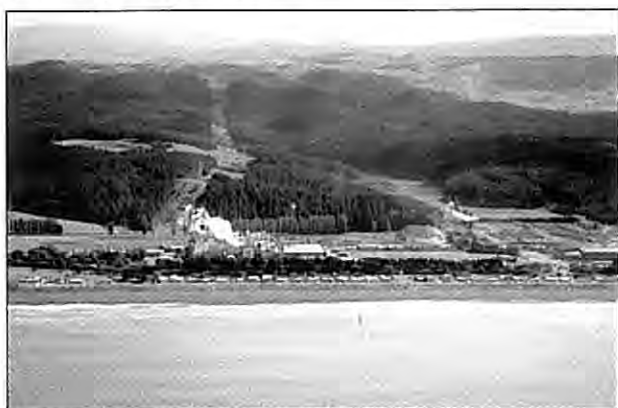
Wairakei Transpower lines at Whirinaki stretching towards the western ranges. (Photo courtesy HBRC)
