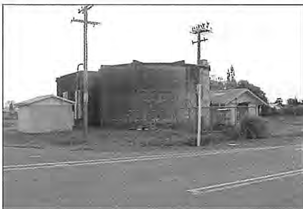
Boundary Reservoirs and pump station at Wairoa (Photo courtesy WDC)
