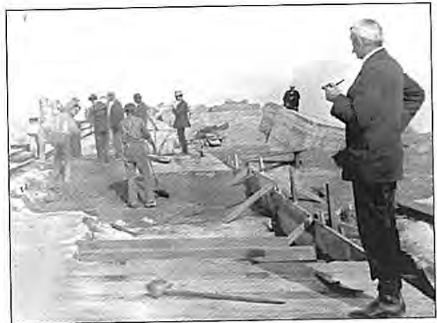
1890's Repairing monoliths on Breakwater after storms
