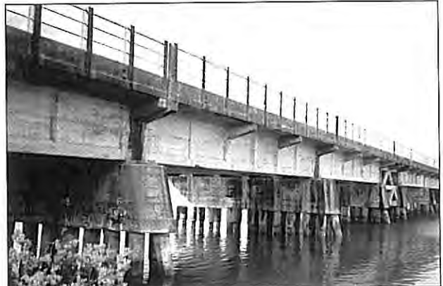
Westshore rail bridge. (Photo courtesy John Keenan)
