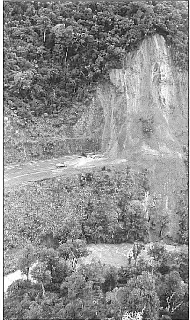
State Highway 5 Runanga landslide 1985. (Photo courtesy of Opus)
