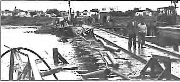
Damage in the Ahuriri Channel caused by the 24 May 1960 tsunami, which struck Napier. The old footbridge linking Napier and Westshore was carried away, damaging gas and water mains and cutting a telephone cable. (Photo courtesy Russell Spiller.)
