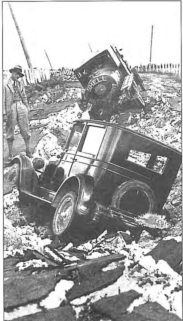
Westshore Embankment Road following 1931 Hawke's Bay Earthquake.
