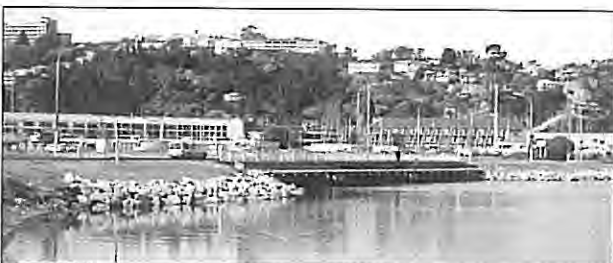
Westshore Bridge on State Highway 2 crosses Aburiri Estuary. (Photo courtesy of Hawke's Bay Regional Council)
