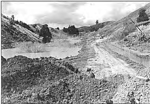
Major landslide Wairoa by Cyclone Bola 1988
