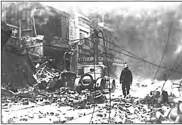
Hastings Street Napier following 1931 Hawke's Bay Earthquake.
