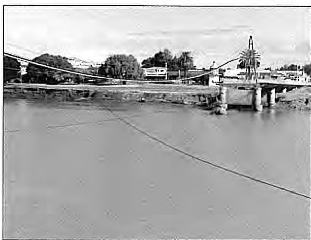
Key Lifeline services, ie water, telephone, electricity and sewerage, straddle Wairoa River after Cyclone Bola 1988.
