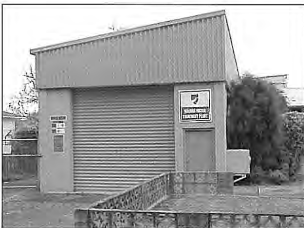
Water treatment plant at Frasertown, Wairoa (Photo courtesy WDC)
