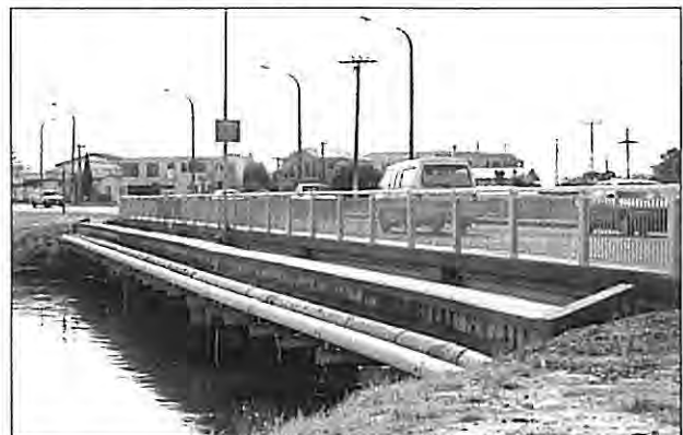
Westshore Bridge on State Highway 2 is a critical lifeline for many utilities. The expressway northern extension when constructed, will mitigate the roading transportation dependence on this structure.
